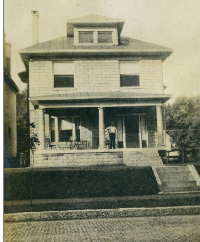
GEORGE BARDIN, STANDS ON THE PORCH OF HIS HOME AT 1050 EVERETT AVE. CIRCA 1912. THERE IS NO HOME AT 1048 AT THIS TIME. A CLOSE UP OF THE SAME PHOTO SHOWS LEADED GLASS WINDOWS IN THE DOOR SIDE LIGHTS IN THE FRONT DOOR. THE NEIGHBORHOOD SHOWS BRICK STREETS AND LIMESTONE CURBS, GRASS IN THE YARD AND ONE SMALL TREE. NO ELECTRICAL WIRES APPEARED IN THE FRONT AT THIS TIME BUT THE POLES AND WIRES SHOW UP IN ALLEY PICTURES AND IN THE FRONT A FEW SHORT YEARS LATER.
