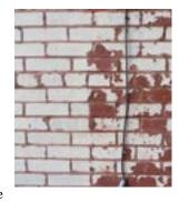
developed, brick was painted to cover dirt. Masonry systems were designed to "breathe." Painting unpainted brick covers existing problems and will result in increased maintenance. Consult with Landmarks staff when planning to repaint masonry that has already been painted.
