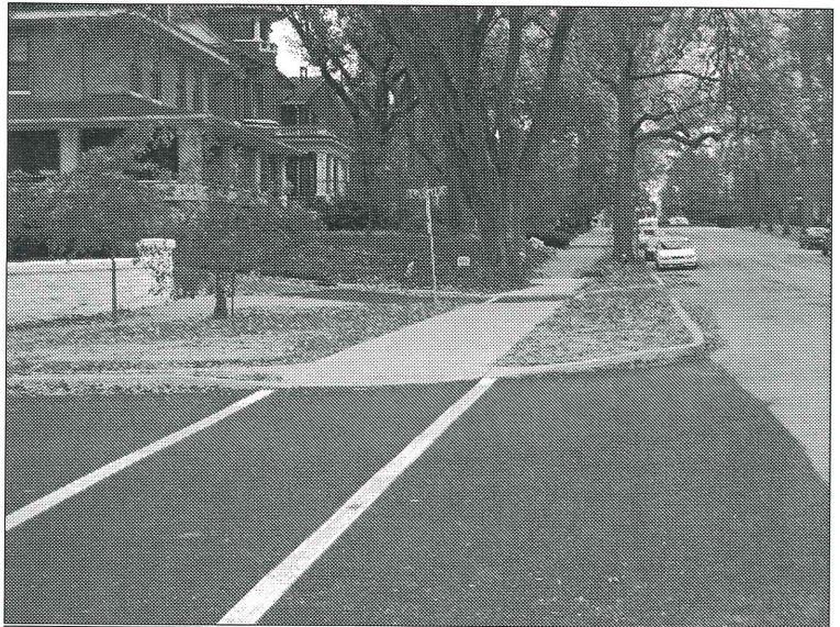
New green space with new sidewalk and pedestrian road striping Photo by Jerry Lyndrup
