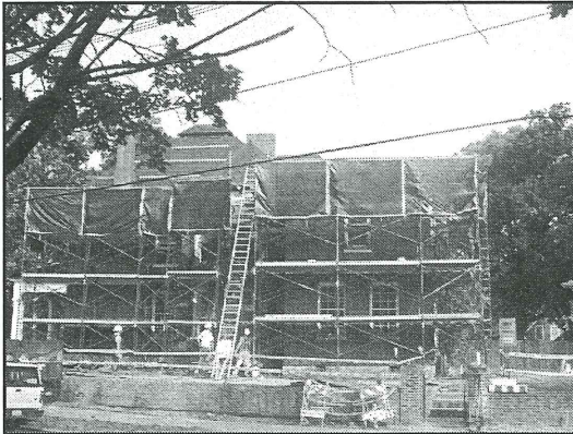
1293 Cherokee Road—view from Longest Avenue Photo by Jerry Grasch
