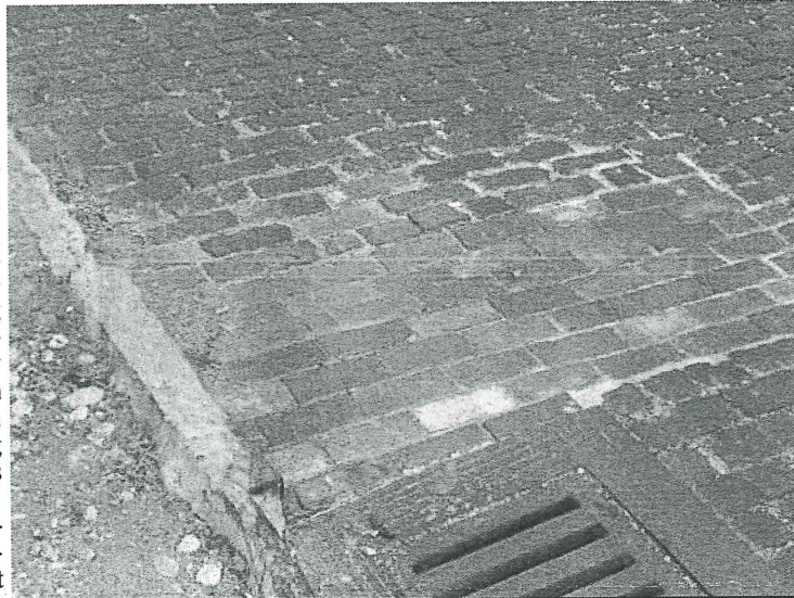
Amy's Repaired Alley (1300 Block between Cherokee Road and Bardstown Road)
