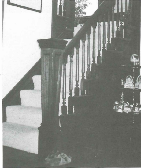
Original staircase with stained woodwork.
